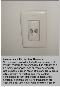
Interior Lighting Vermont building energy codes allow for 1.1 watts/sf for lighting. Through the use of T-8 fluorescent fixtures this project accomplished lighting efficiencies of 0.72 watts/sf on the 2nd floor and 0.81 watts/sf on the 1st floor. Therefore, as a total building project, interior lighting consumes 30% less energy than code permits.
