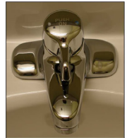
Auto Faucets Auto control faucets contribute to water conservation for the building by only providing water when hands are in the sink. Auto control faucets also limit the spread of germs and lead to a cleaner bathroom habitat for all building occupants.
