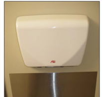
Hand Dryers Air drying of hands significantly reduces the amount of paper waste in the building which results in a 70% reduction in CO2 emissions due to from the reduced manufacturing of paper towels.
