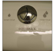
Dual Flush Toilets Dual flush toilets contribute to water savings by providing two buttons to operate the flush. One button provides a short 0.8 gallon flush while the second button provides a full 1.6 gallon flush.
